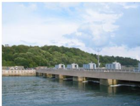
Barrage of the tidal power plant on the estuary of the Rance River in Bretagne, France
